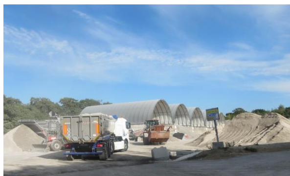
Eco-site – La Croix Irtelle
